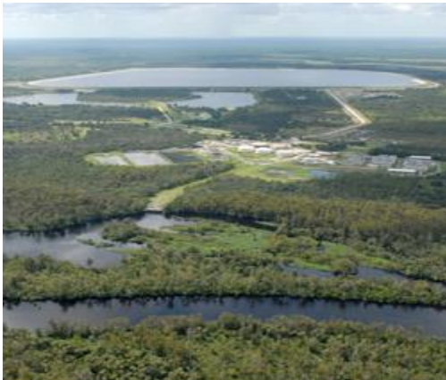
Figure 1. Peace River Treatment Facility
