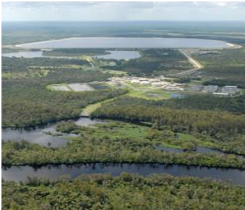
Figure 1. Peace River Treatment Facility
